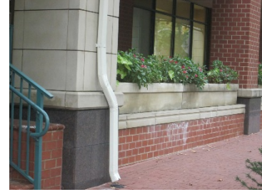
Window planters such as these can provide a limited protection from window breakage by making it more difficult for a person at street level to swing an object at the window with any amount of force.
